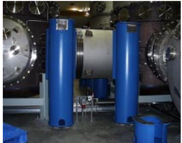
Figure 5 BSC seismic isolation system support piers, LHO
