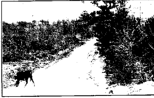
preparation and road preparation work in the rural area north of Livingston.
