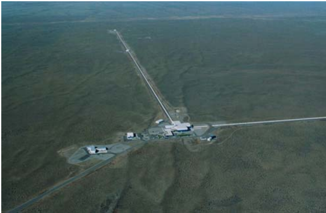
Figure 1: Aerial photograph of the LIGO Hanford Observatory. View is looking towards the SW, along the Y-arm. Two buildings are visible: one is at the 2 km midpoint; the other is at the 4 km terminus of the arm. The white structures along the arms are concrete covers protecting the vacuum tube.
